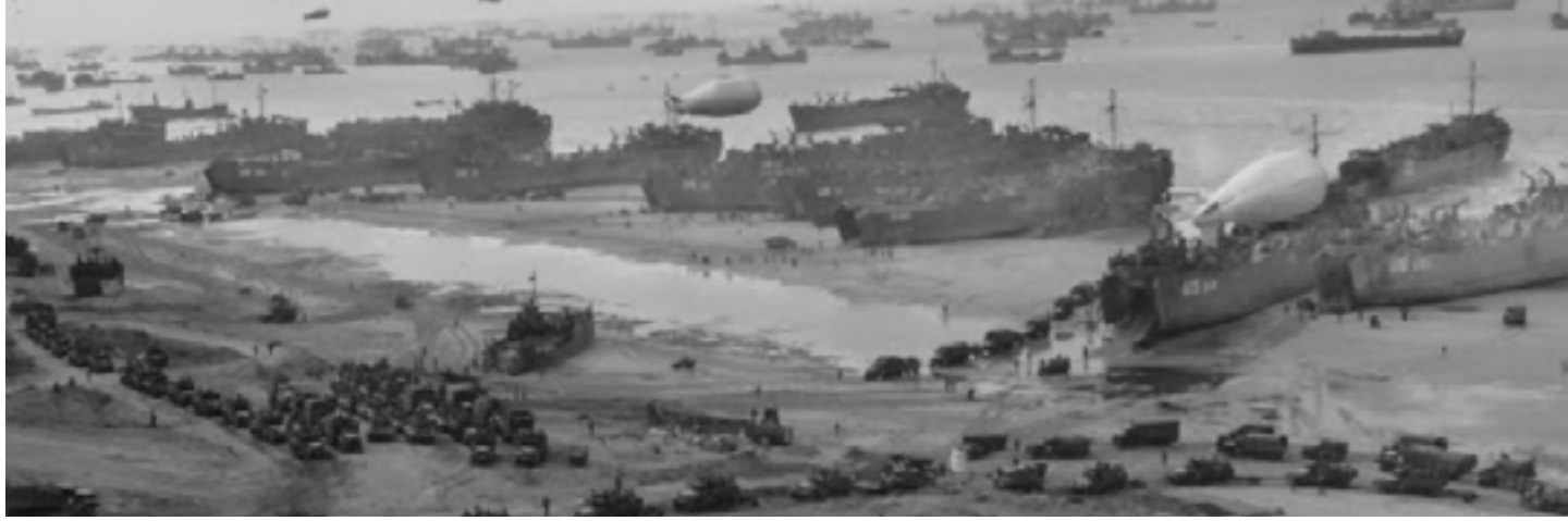
PHOTO NATIONAL ARCHIVES AND RECORDS ADMINISTRATION, U.S. NATIONAL ARCHIVES (06-06-1944)
